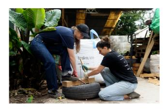
To avoid the waste of these elements, -which are normally burnt to litter-, we are using tyres as foundations to protect the timber from capillarity. Tyres may also be used as design components, bolting them by the sides -as the middle ring contains metal wires-, although their thermal qualities must be considered.
